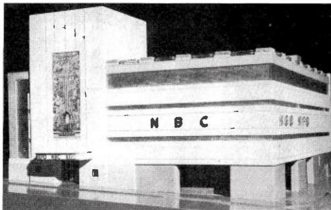
ARCHITECT'S scale model of the much-heralded NBC building in San Francisco showing the building costing over a million dollars which will house studios and technical equipment for KGO and KPO. Five stories high, it is constructed of reinforced concrete, trimmed with bands of translucent glass brick. There are no windows, the structure being air conditioned throughout. The building will provide 52,800 square feet of floor space, more than double the present quarters.
